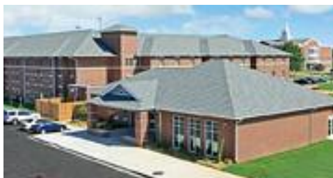
➤ The RSU University Village B apartments are 87,118-square-feet and can house 255 students. This complex features wireless Internet, a clubhouse, and meeting rooms.
