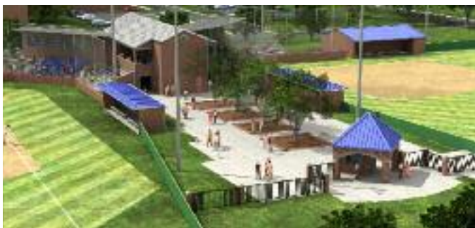
The new baseball/softball facility will include concessions, restrooms, grandstands and a ticket booth with a paved entry plaza.
