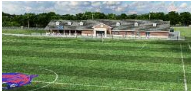
The Soldier Field renovation includes artificial turf, locker rooms and training facilities for soccer and cross country, as well as, concession stand and public restrooms.
